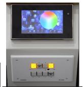
Touch panels to remotely power-up amp racks, console and for room lighting control
